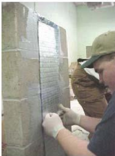
(c) Installation of Fibers
