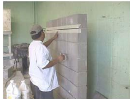
(b) Masking of Masonry
