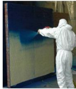
Spraying the second layer of polyurea over the grid
