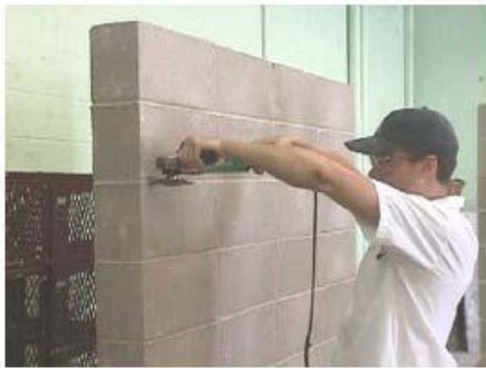
(a) Grinding of Joints
