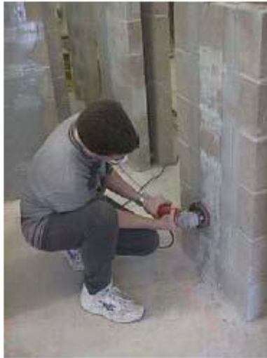
(a) Leveling of Surface
