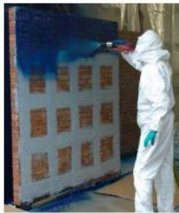
Spraying polyurea over the strengthening layer
