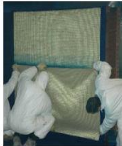
Laying down the grid over the first layer of polyurea
